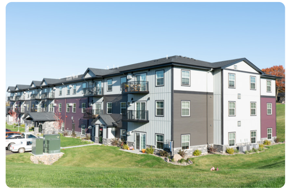
Long Prairie apartment building with CTC's fiber-to-the-unit (new construction).
